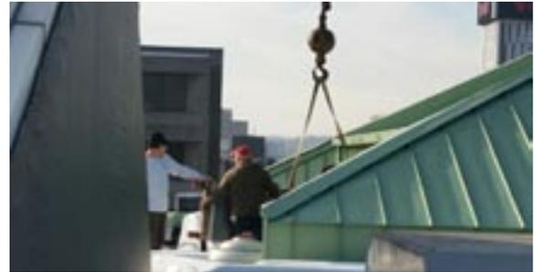
*The scope of the work being done on the 1985 Butler addition is the removal of the two existing DX cooling condensing units from the rooftop. Piping has been added to the existing air handlers from the new chiller recently installed. There will be two replacement cooling coils installed in the air handling units cooling the executive offices, business offices, 2nd floor balcony, Beecher Court, shipping and receiving, two Mesaros Galleries, offices and the education gallery in the lower level.*
